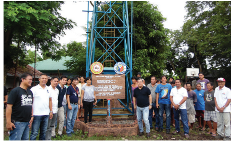
Opening of Purok Narra Water Supply System Level III at Barangay Malingin last August 1 attended by City and Malingin Officials.
